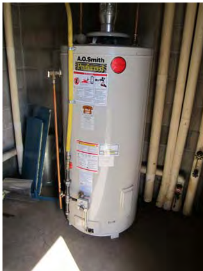
Concurrent with boiler replacement has been the installation of freestanding tanks for production of domestic hot water
