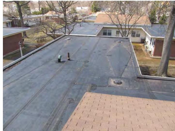
Adhered membrane and three-tab shingle roof coverings are in good condition
