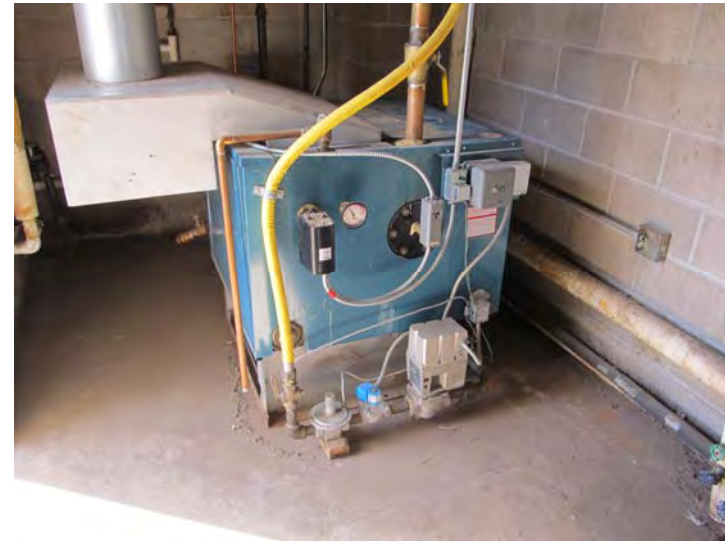
Two residential buildings feature central boilers that have been replaced in recent years
