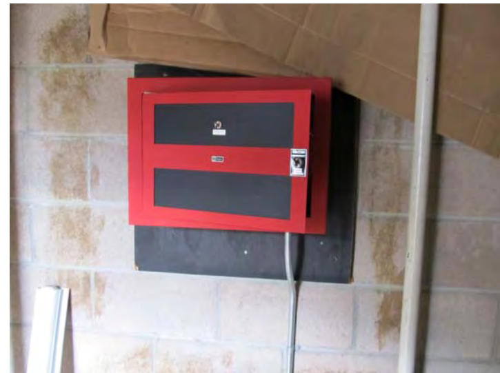
Typical older fire alarm control panel found at each building
