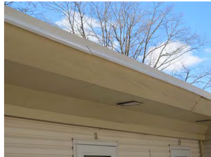
Painted wood soffits and fascias are in need of repair and painting in the near-term
