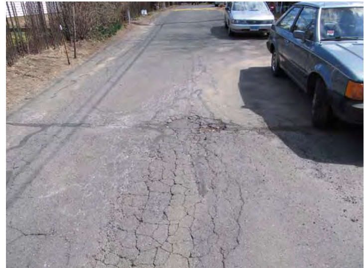
Asphalt paving exhibits cracks and age-related wear
