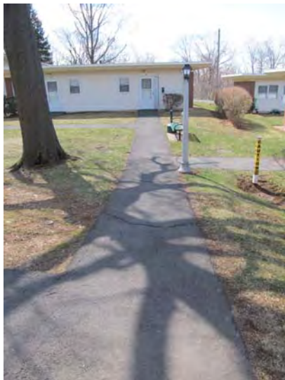
Asphalt walkways also exhibit cracks and wear
