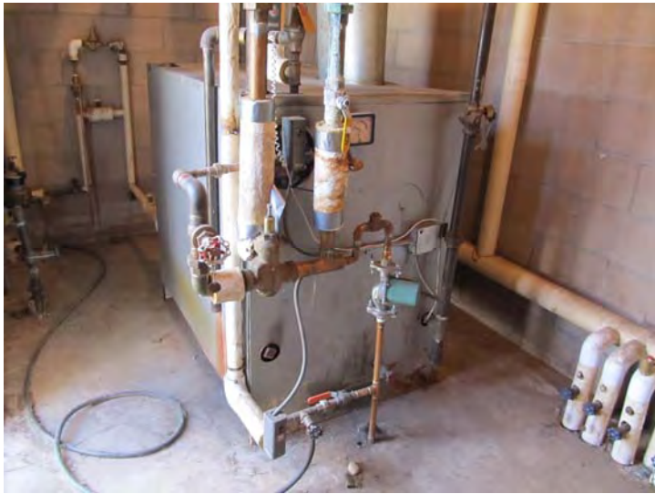
Typical older central boiler with an internal heat exchanger for domestic hot water generation at a residential building
