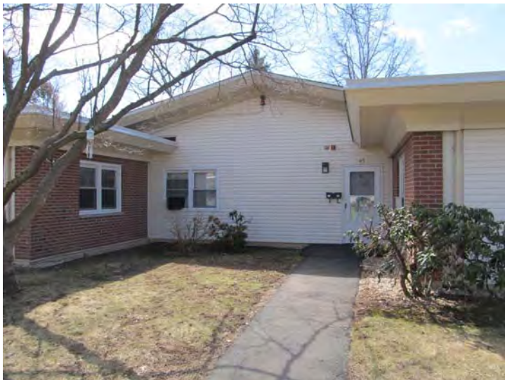
Brick veneer and vinyl siding exterior wall finishes in generally good condition at the present time
